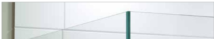
UV Bonding (Two pieces of glass bonded together).
